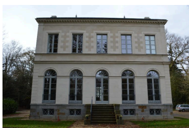
Façade principale Phot. Maïlys Provost IVR53_20183505952NUCA
