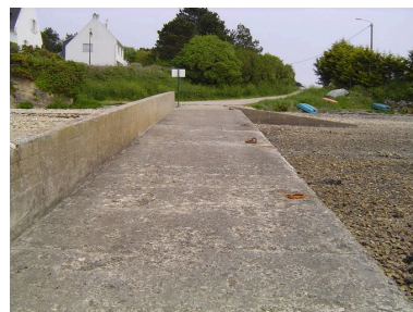
Cale de Rostellec Phot. Clotilde Buhot IVR53_20062908527NUCA
