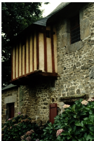
Logis, façade postérieure, latrines. Phot. Guy Artur, Phot. Norbert Lambart IVR53_19853500447ZA
