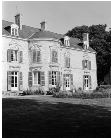
Elévation est, partie nord. Phot. Guy Artur, Phot. Norbert Lambart IVR53_19915600860X
