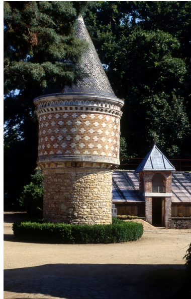
Colombier Phot. Guy Artur, Phot. Norbert Lambart IVR53_19915601002ZA
