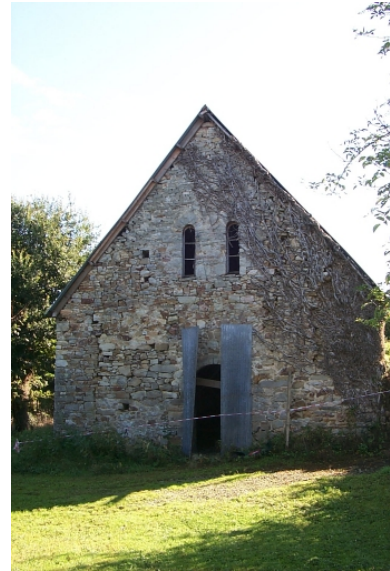
Elévation ouest Phot. Xavier Gilbert IVR53_20013509861NUCA
