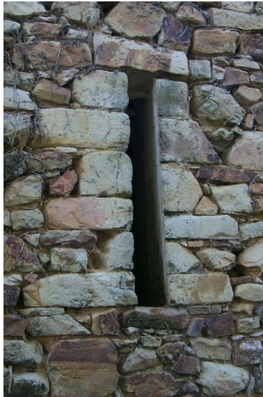
Nef, mur nord, baie Phot. Xavier Gilbert IVR53_20013509860NUCA
