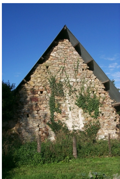
Chevet Phot. Xavier Gilbert IVR53_20013509856NUCA
