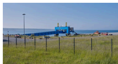
Passerelle Ro-ro Phot. Bernard Bègne IVR53_20232900354NUCA
