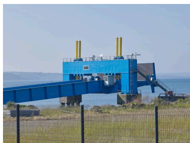
Passerelle Ro-ro Phot. Bernard Bègne IVR53_20232900355NUCA
