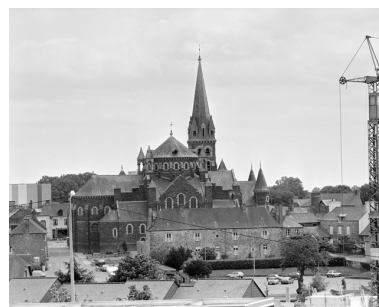
Vue de situation nord Phot. Guy Artur, Phot. Norbert Lambart IVR53_19943501055X
