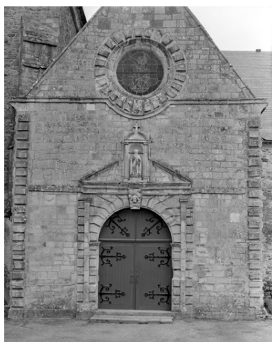
Elévation ouest Repro. Guy Artur, Repro. Norbert Lambart IVR53_19943501512XB
