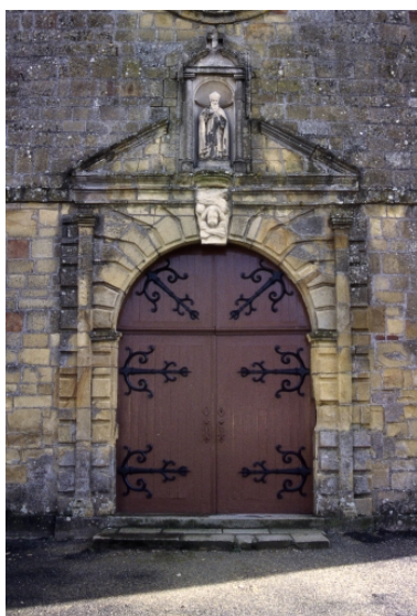
Portail ouest Phot. Guy Artur, Phot. Norbert Lambart IVR53_19943502740XA
