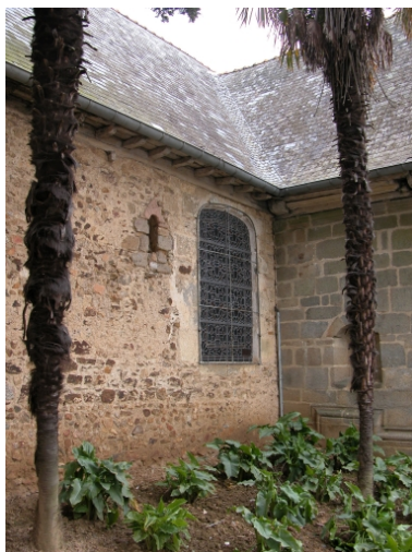
Mur sud Phot. Claude Quillivic IVR53_20043503056NUCA
