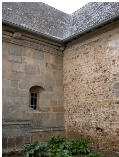
Mur sud Phot. Claude Quillivic IVR53_20043503055NUCA
