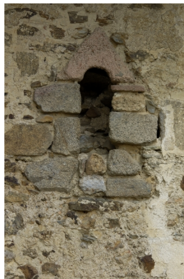
Baie romane Phot. Bernard Bègne IVR53_20043500910NUCA
