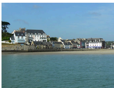
Front portuaire de Morgat Phot. Johan Vincent IVR53_20072908748NUCA
