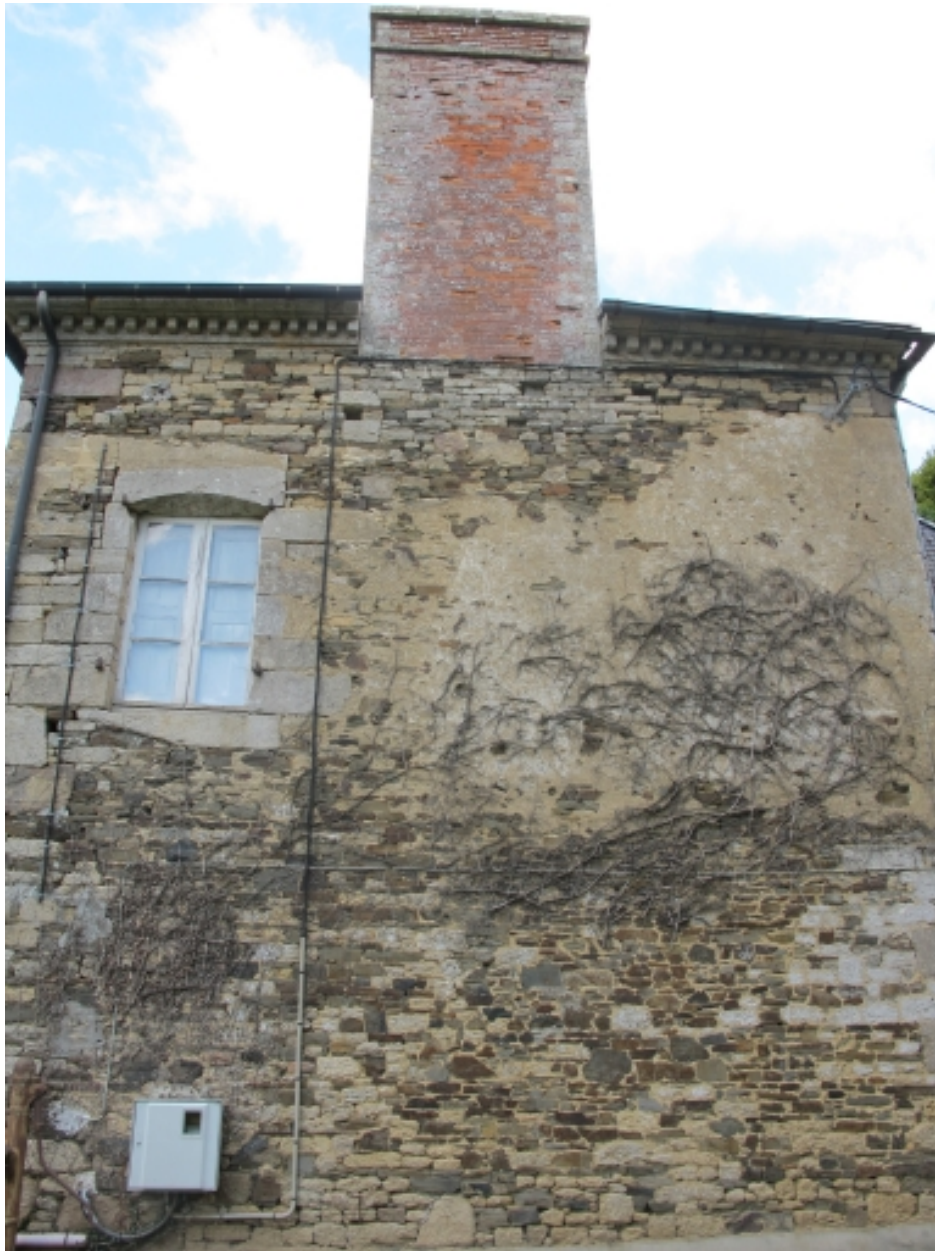
Logis, pignon sud
