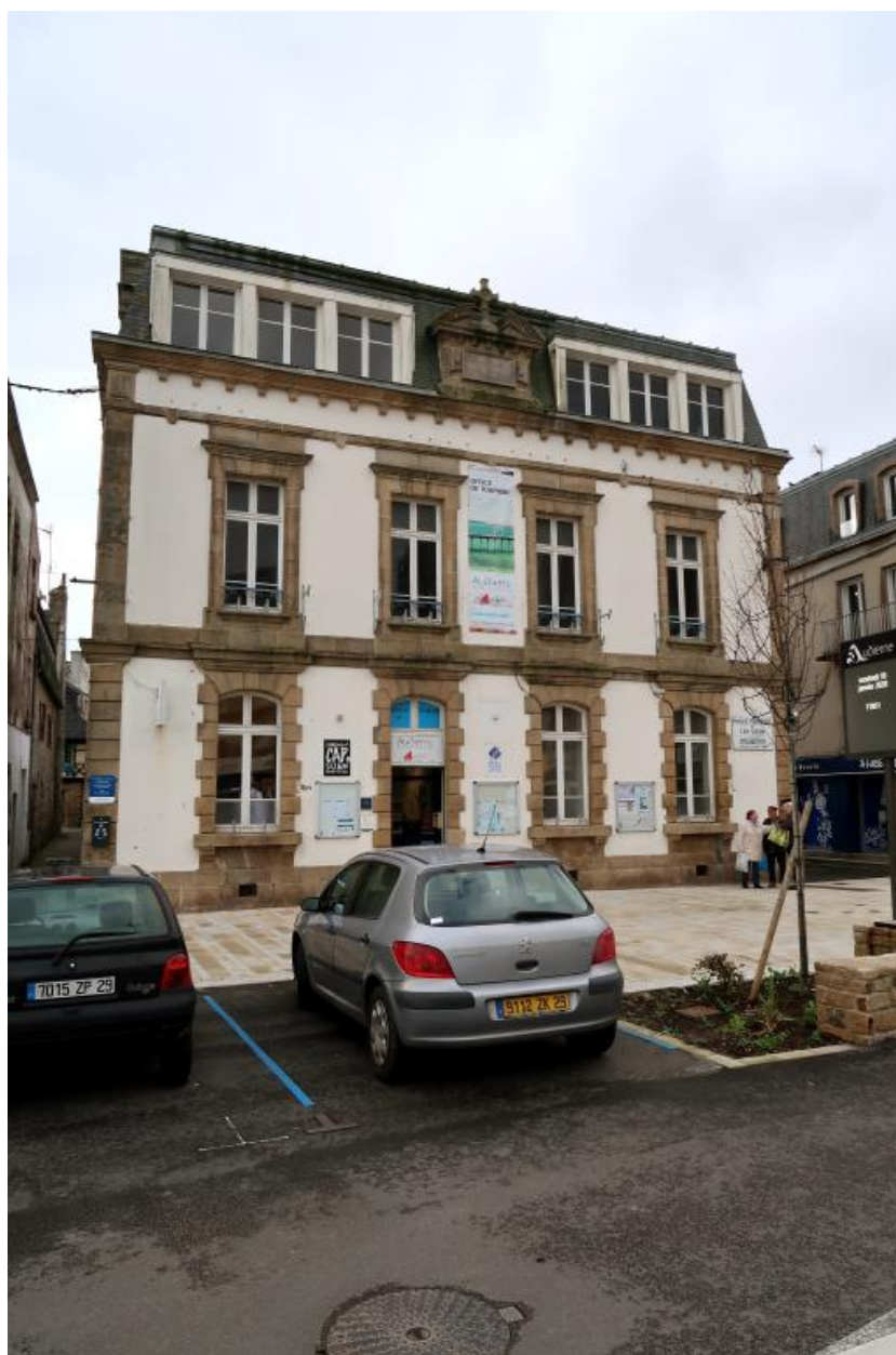
Pavillon est, élévation antérieure est. (2020)
