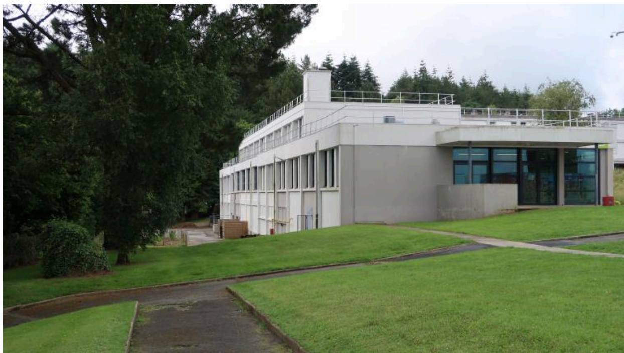
Bâtiment B (restauration), façade est.
