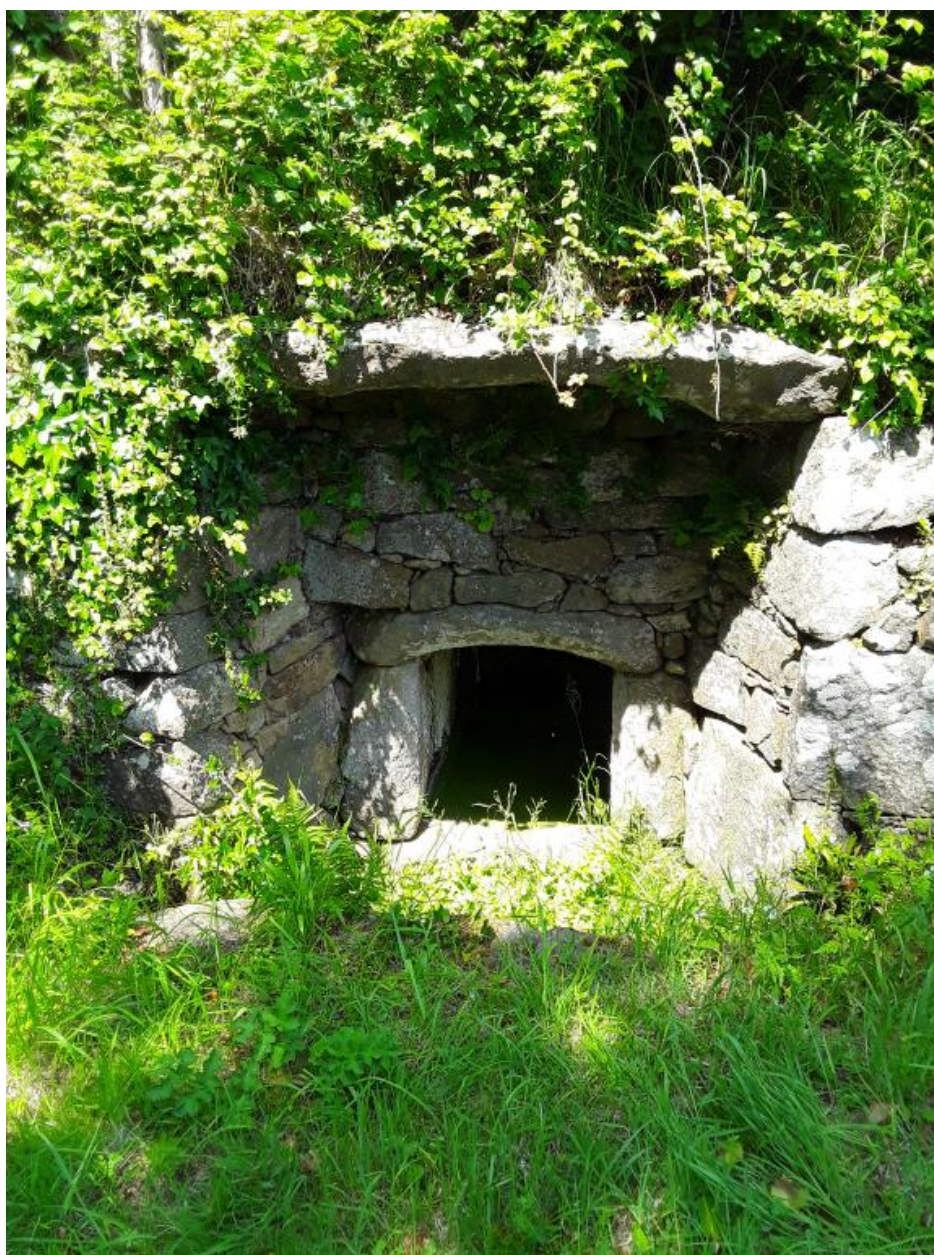
Fontaine-mur de Kergaradec. (2018)
