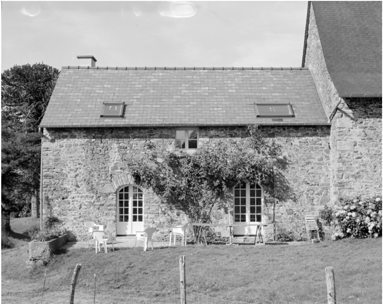
Logis, élévation est.
