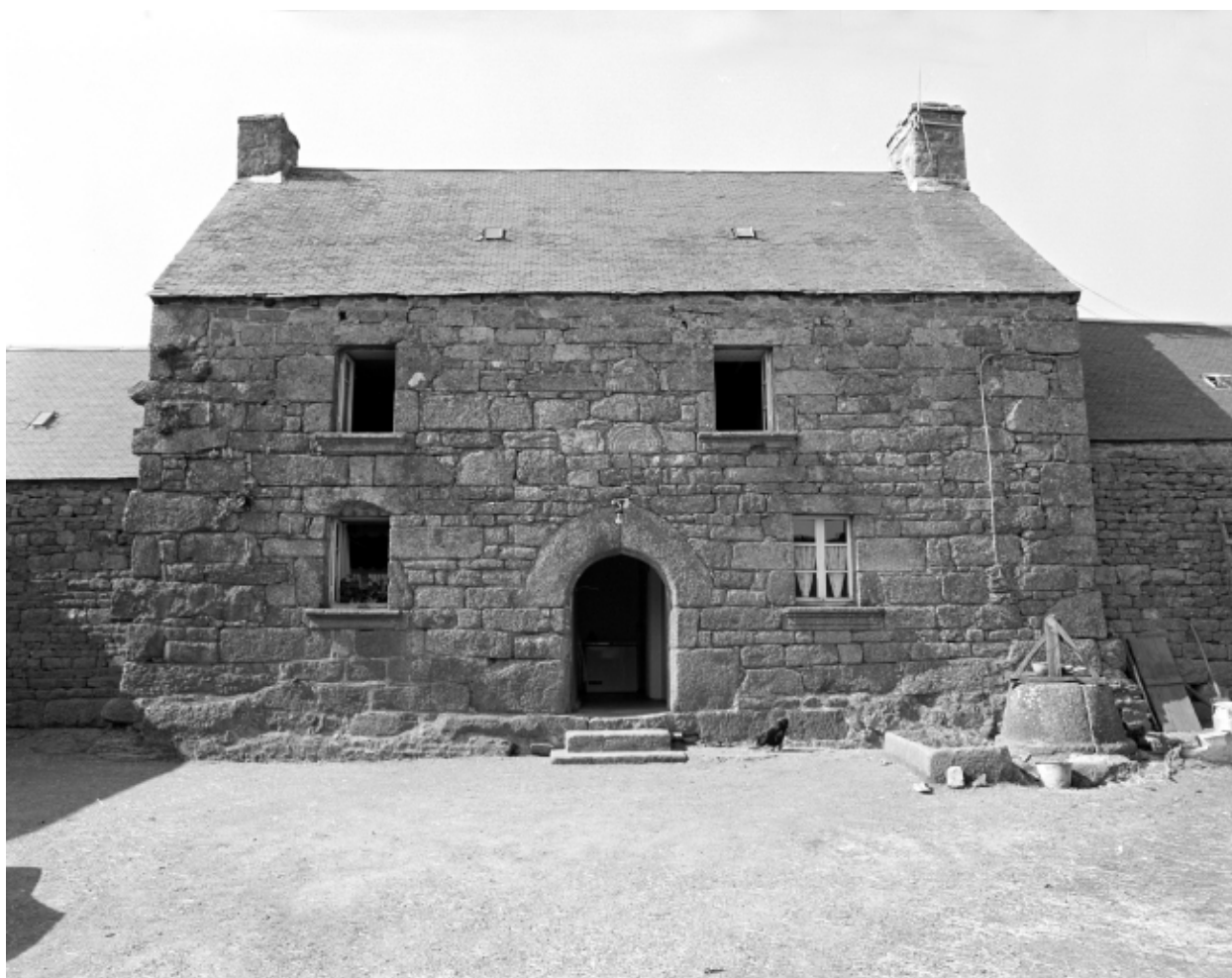
Logis, façade sud
