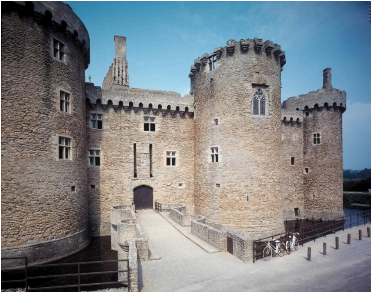
Château fort, logis est, élévation est.
