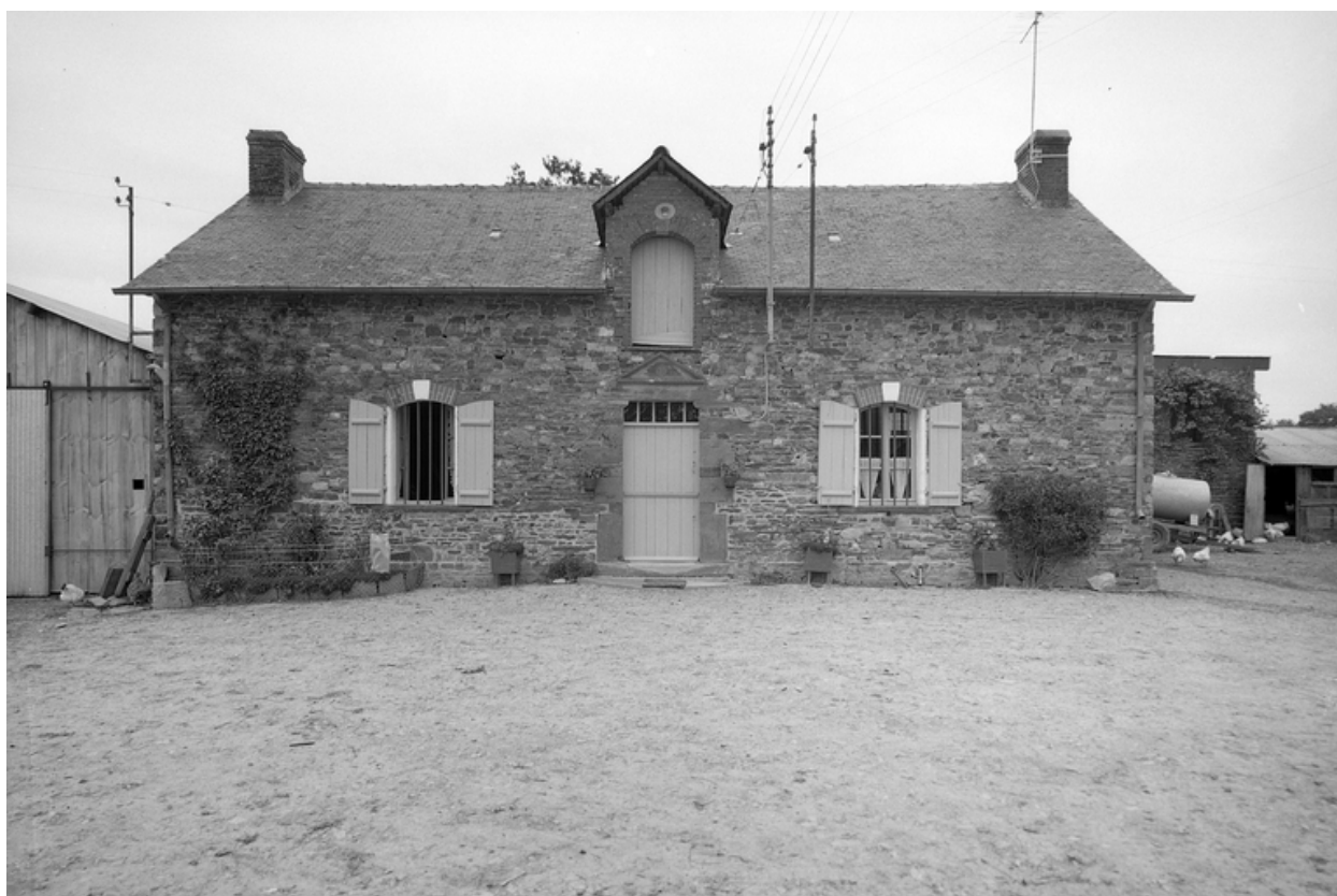
Logis, façade sud.
