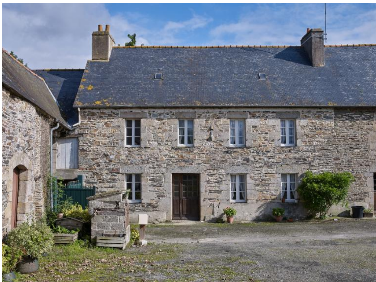
Logis 1831. Elévation sud
