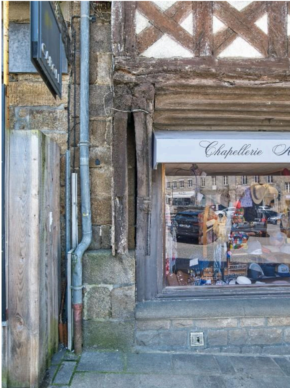
Double poteau soutenant la solive de rive.
