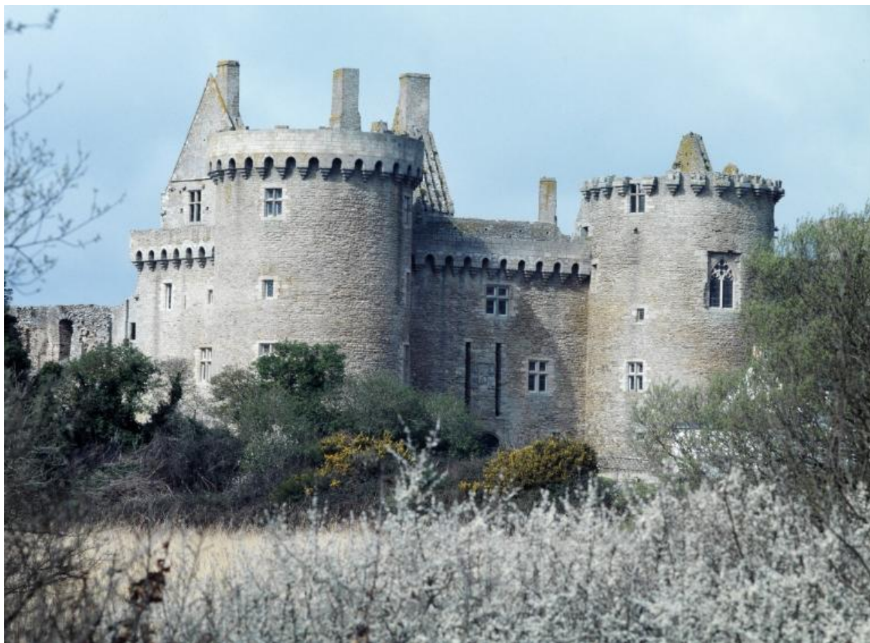
Château fort, logis est, élévation est.
