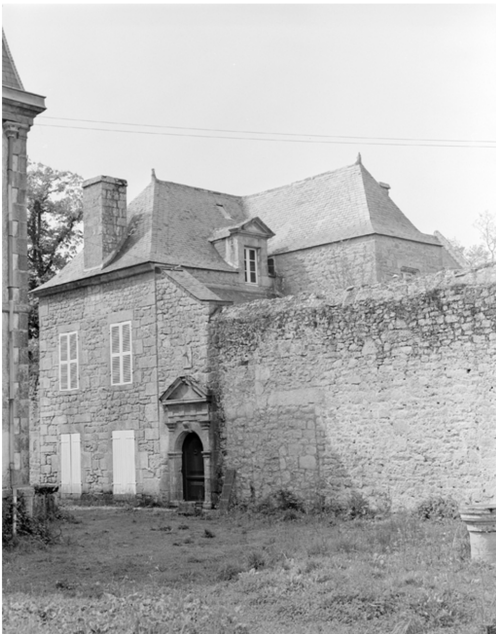
Logis abbatial, élévation sud. (1983)
